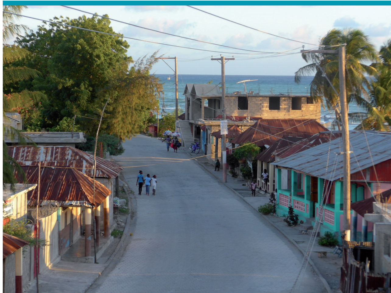
In Haiti, 19 US-based electric co-operatives and 37 volunteer linemen worked with the National Rural Electric Co-operative Association (NRECA) International to help build Haiti's first electric co-operative. The possibilities are now endless for three towns in the southwestern region of the country, because a better life starts with power.
